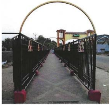
The Welcoming Village Entrance Gate
